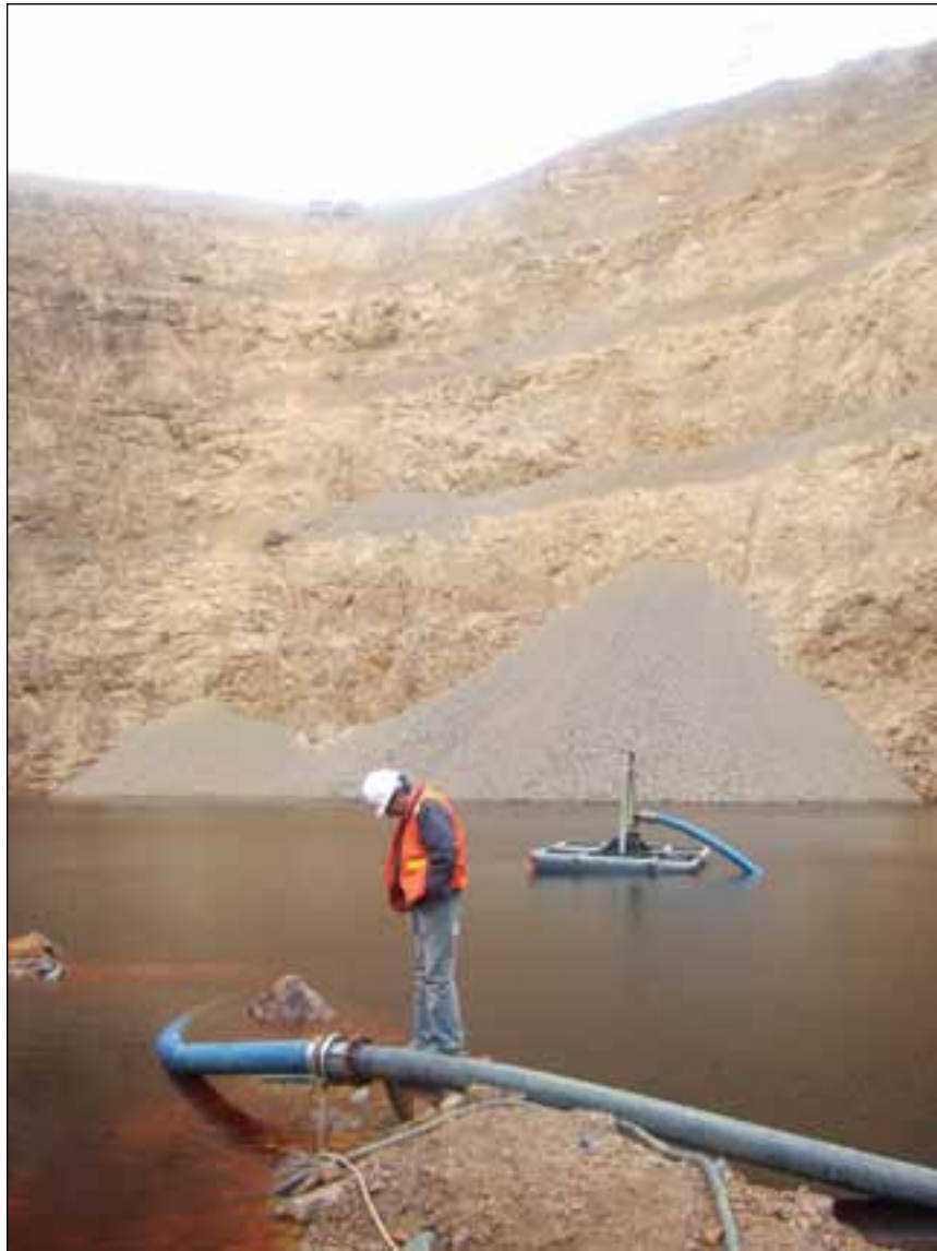
Dewatering collection pits
