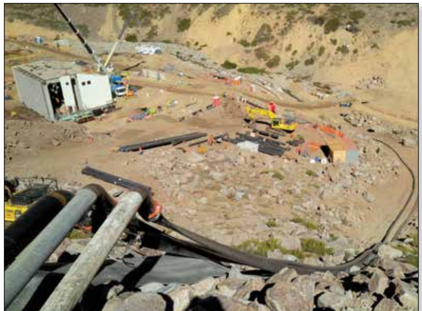
High pressure dewatering
