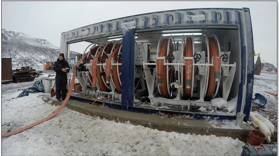
FUEL FLEX Hose Reel Systems can be housed in a converted and insulated, temperature controlled, sea container.
